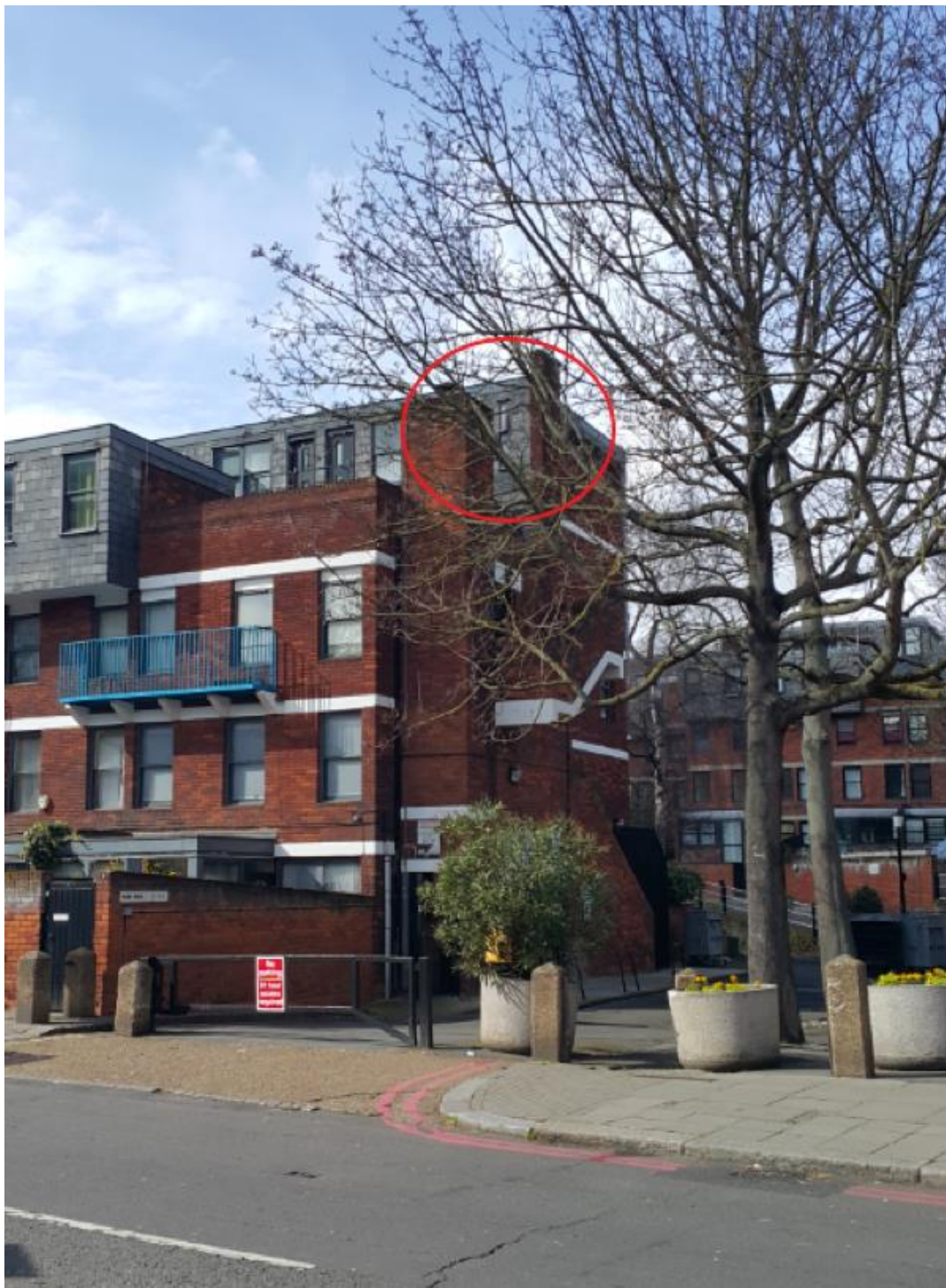
Photograph from Rampayne Street (window location identified)
